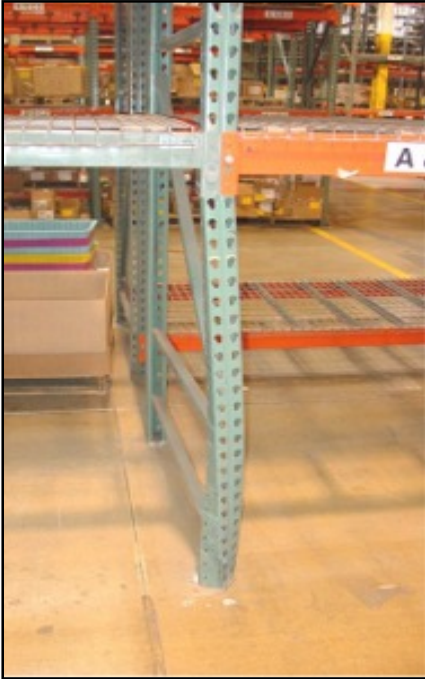
Damaged Frame
